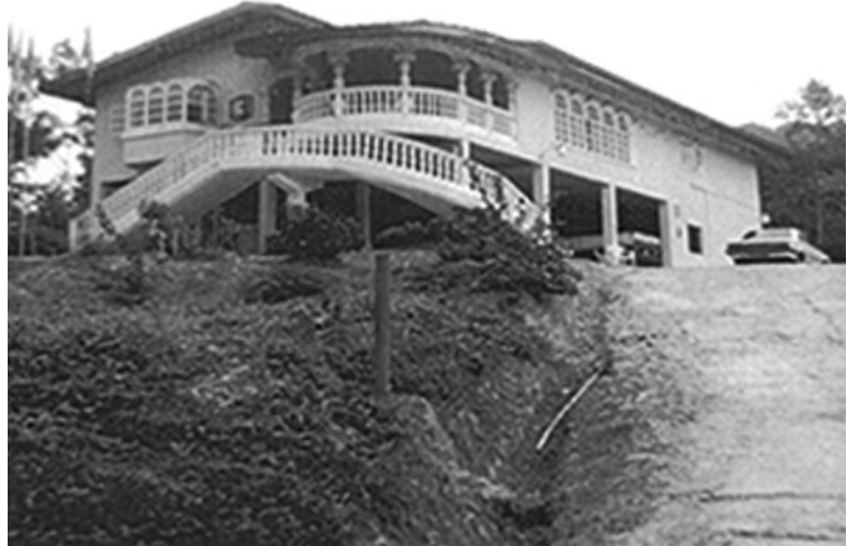
Fig. 1: Indo-Trinidadian big house with balustraded staircase and gallery and metal Om sign on the façade to indicate the owners Hindu affiliation. (Photo Credit: Wahab)
